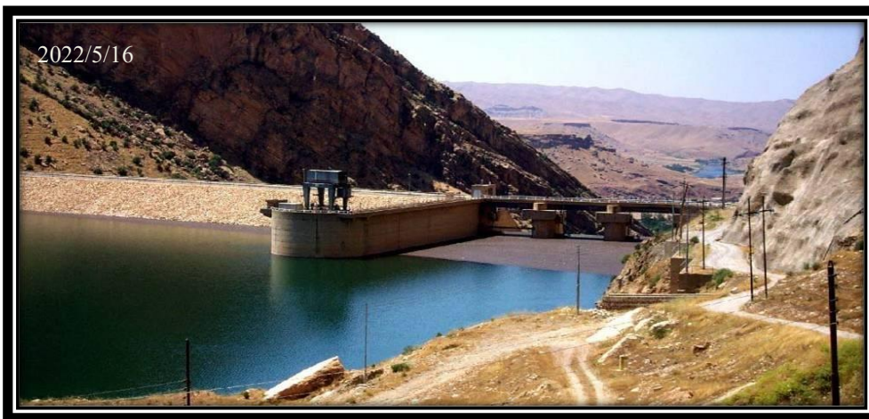
Figure 6. Darbandikhan Lake before the dam for the year 2022 Field study in 16-5-202
